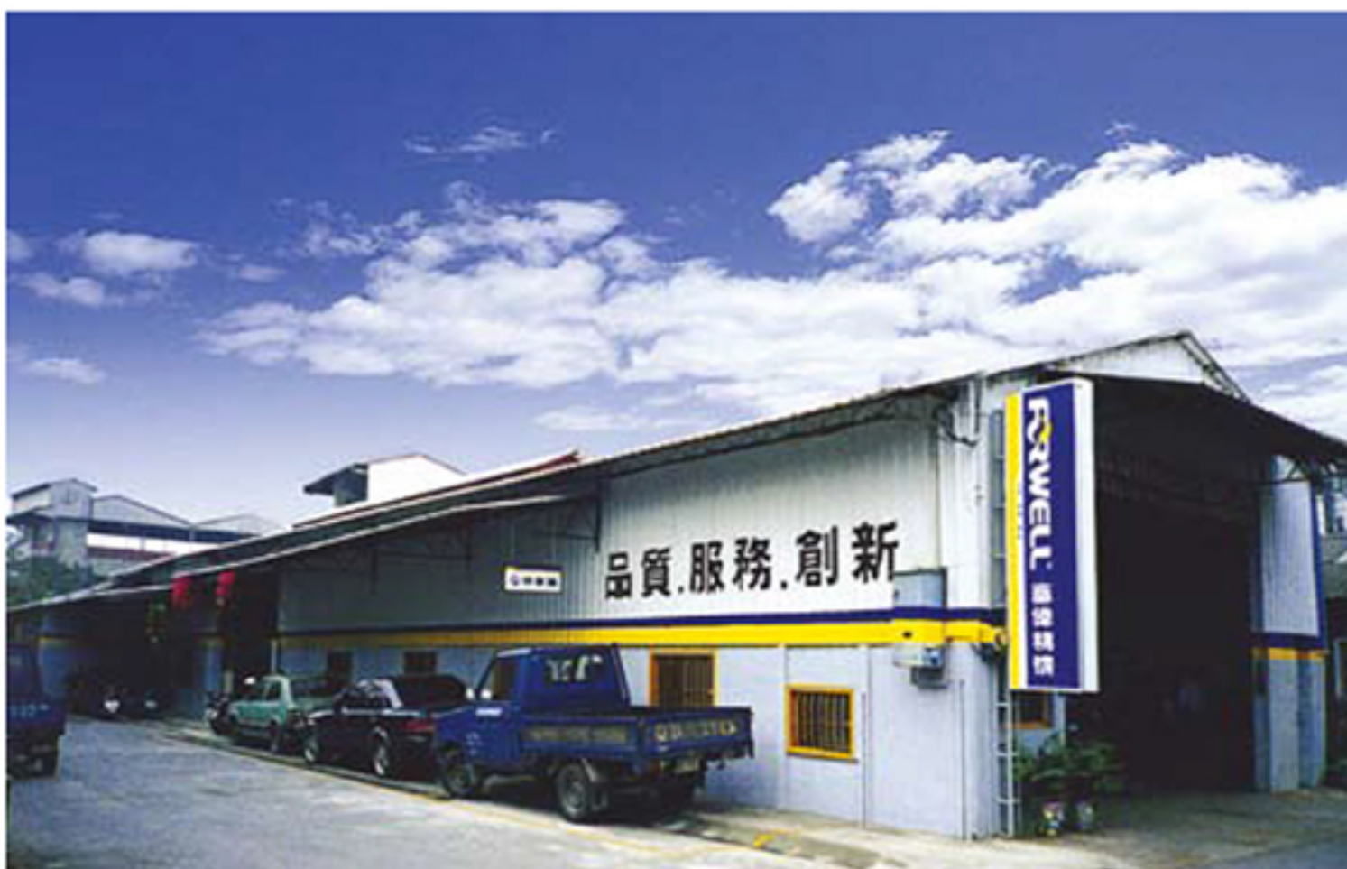
廠房外觀 Outward appearance of the factory
